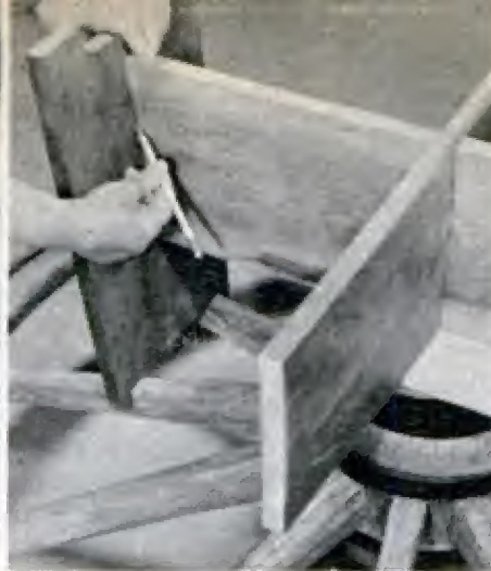
EACH LEG is marked, drilled and attached to cross brace individually to assure its proper location
